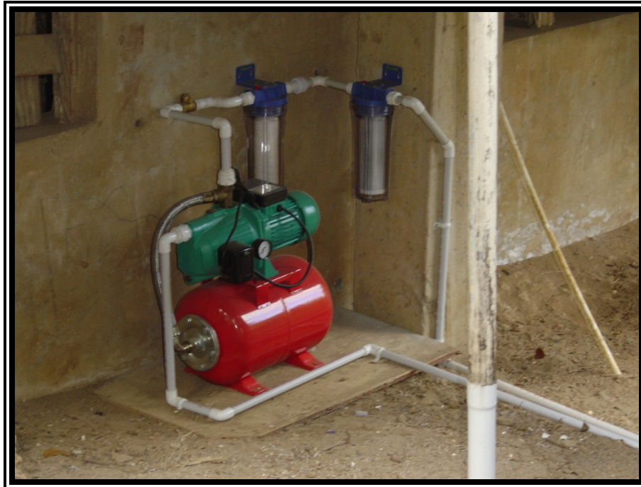
Figure 8 – Installation of charcoal filter and fabric filter at residential home
